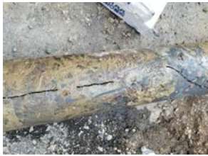
Broken pipe removed and replaced on SW Garden View.
